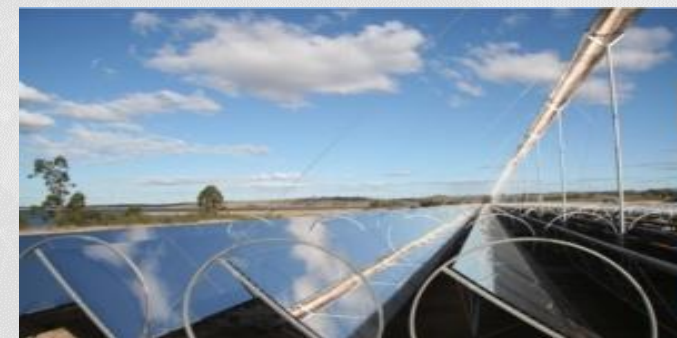
Fresnel: Kimberlina Solar Thermal Energy Plant - 5 MW , Bakersfield - California
