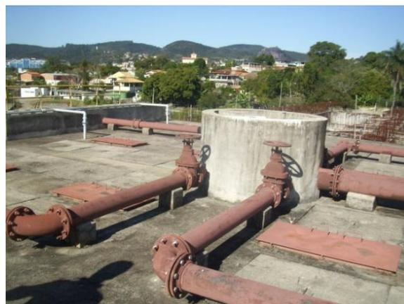
Figura 4.4 – Reator UASB da ETE Principal
